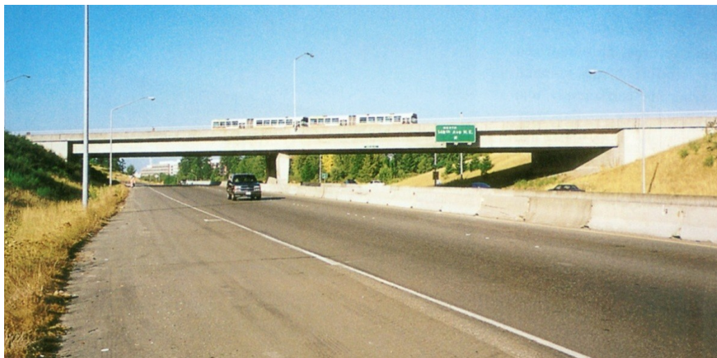
Figure C17- Two-span semi-integral abutment bridge with an overall length of 89 m, width of 11.6 m, and a skew angle of 45^\circ (Nicholson, Barr, Cooke, Hickman, Jones and Taylor, 1997).
