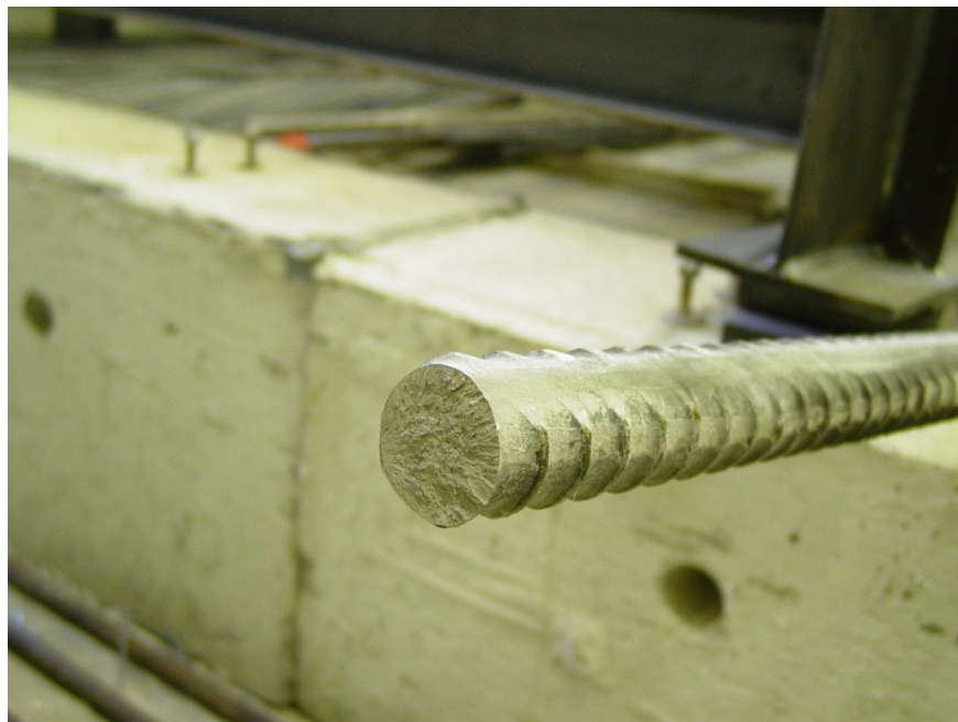
Figure 4-36- Failure of the dywidag
