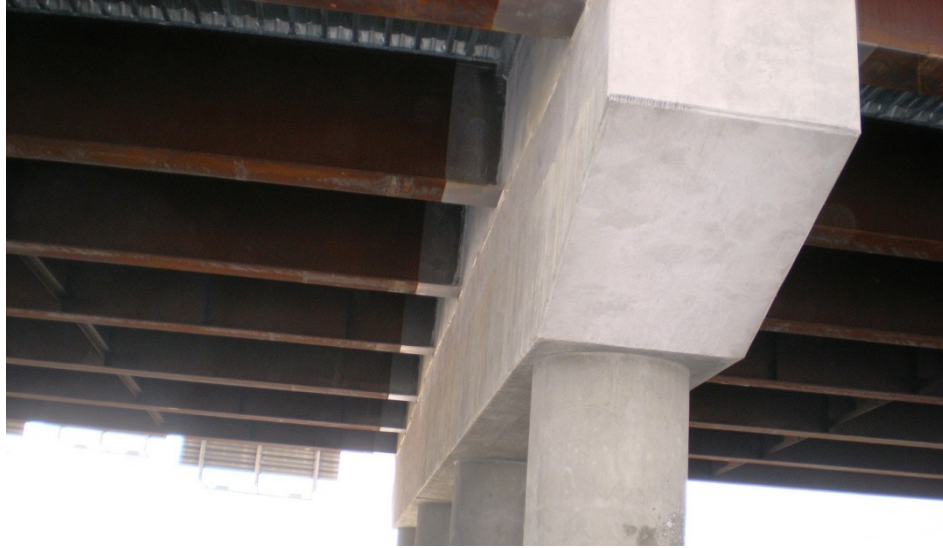
Figure C49- Integral cap as completed
