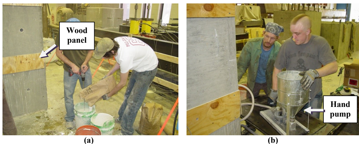
Figure 4-20- (a) preparing fresh hydrostone (b) pumping the hydrostone into the gaps
