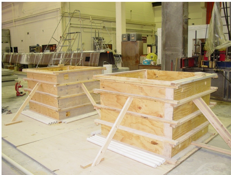
Figure 4-9- Casts for the caps
