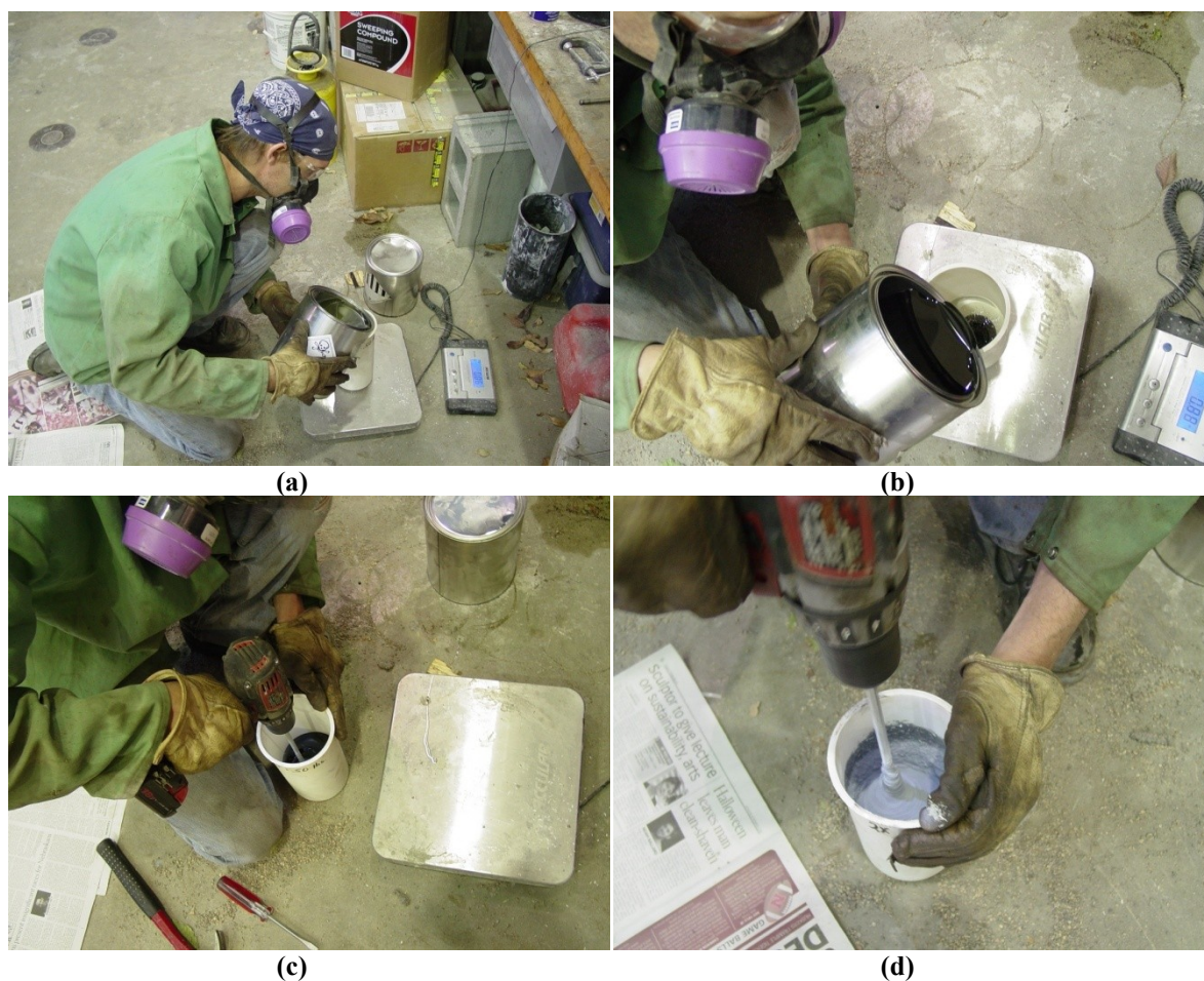
Figure 4-66- Delpatch mixing procedure
