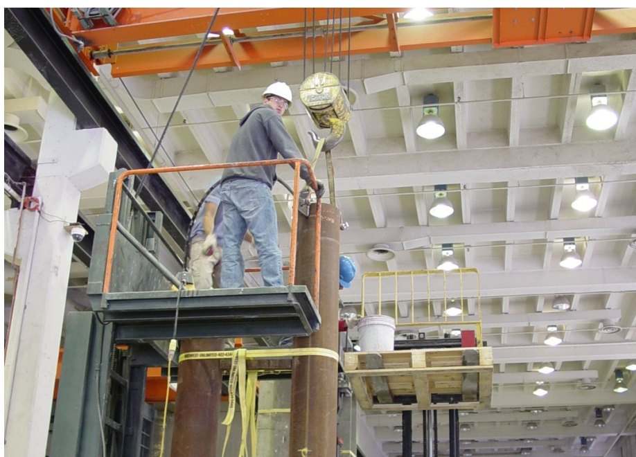
Figure 4-12- Pouring concrete into the pipe
