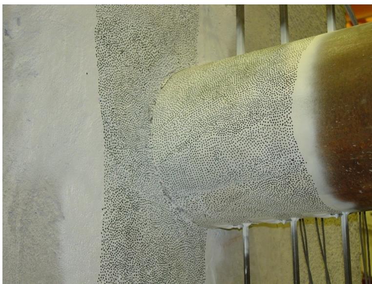
Figure 4-23- Condition of the connection at load stage 3-8 ( \pm 2.00 in)
