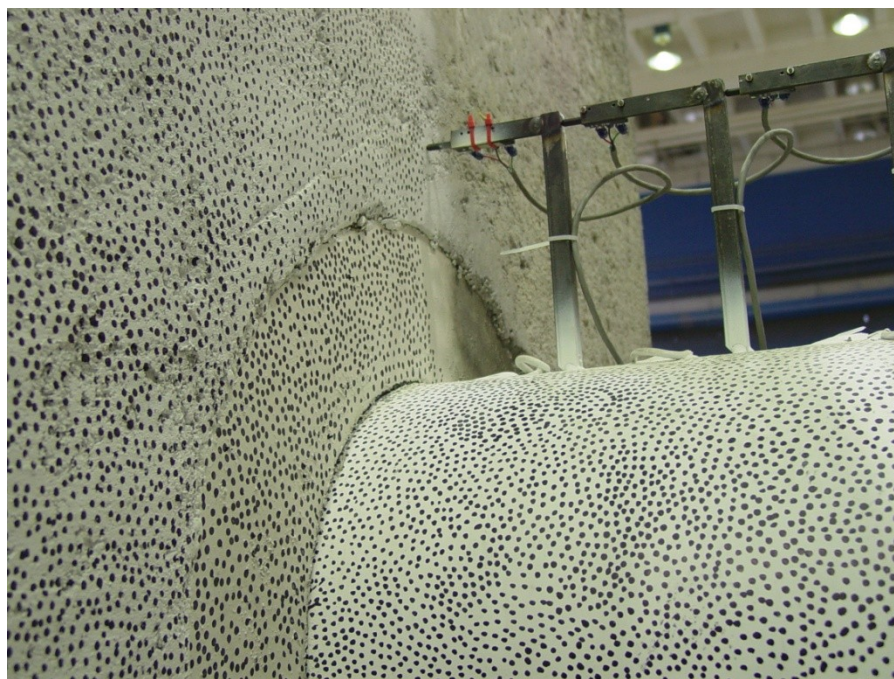
Figure 4-29- Condition of the connection at stage 1-9 ( \pm 2.00 in)
