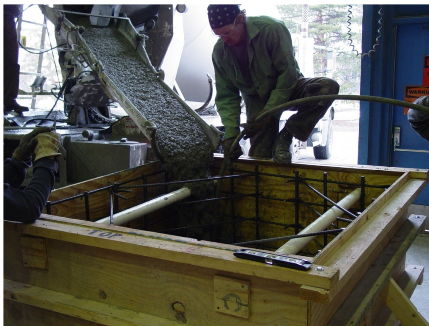
Figure 4-13- First pour into Specimen #2
