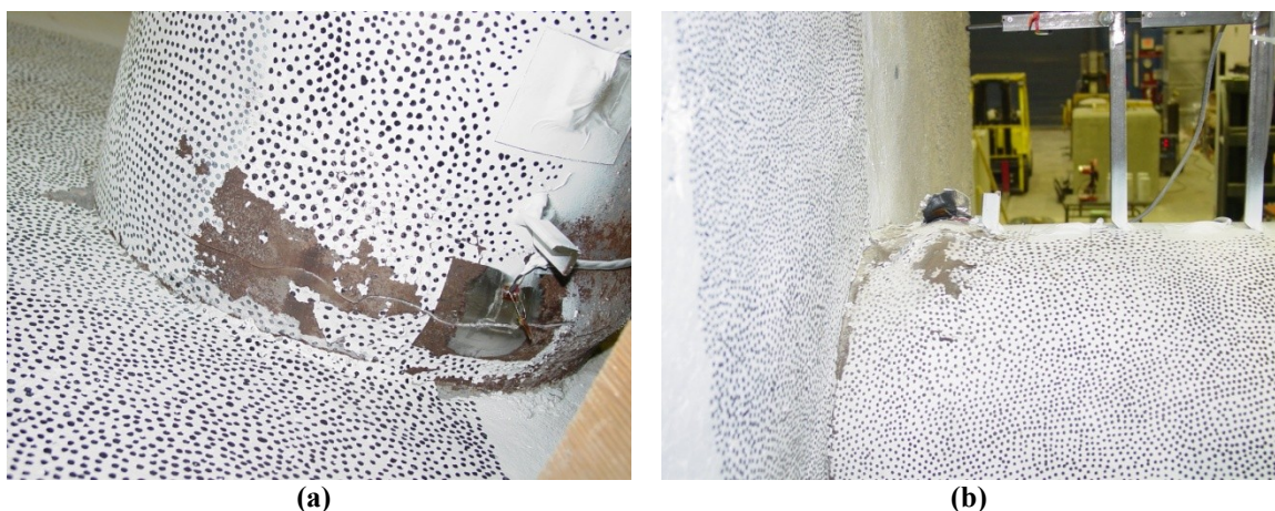
Figure 4-26- Condition of connection at load stage 3-18 ( \pm 4.50 in) (a) huge crack at the bottom (b) large deformation at the top
